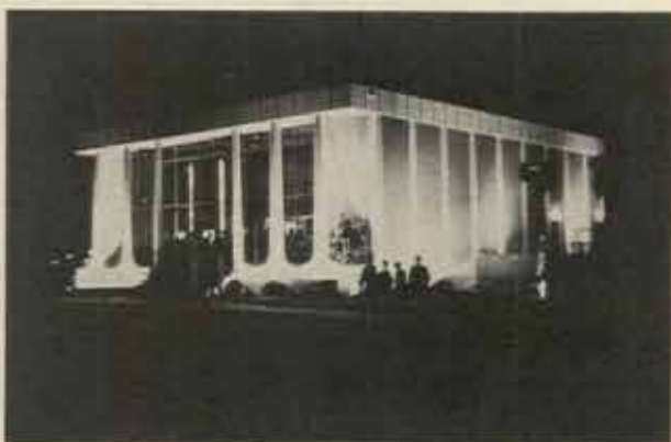
NIGHT LIGHTING makes impressive sales office a 24-hour advertisement for the Showcase and for Hallcraft Homes.
